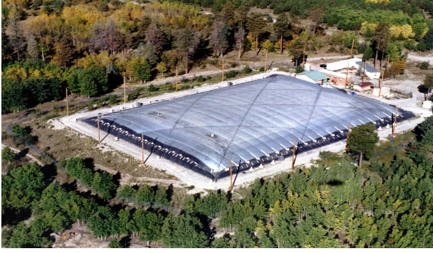
Figure 1: Aerial view of the Milagro pond with the light-tight cover inflated for work inside.
