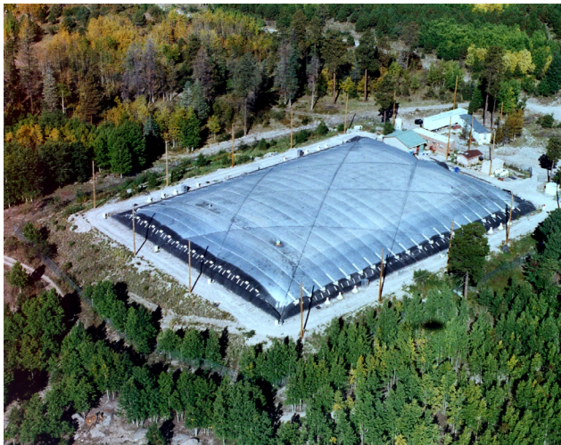
Figure 1 Aerial view of the Milagro Gamma-Ray Observatory site. Visible are the large covered pond (foreground) and the counting house, pond utility building, and access roads (background)
