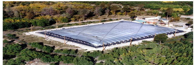
Fig. 1. Aerial view of the Milagro pond with the light-tight cover inflated for work inside..
