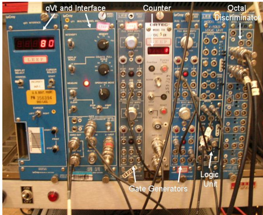
FIGURE 4: NIM BIN ELECTRONICS
